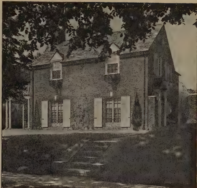
645 Dwight James Baum, architect; photograph by John Wallace Gillies
